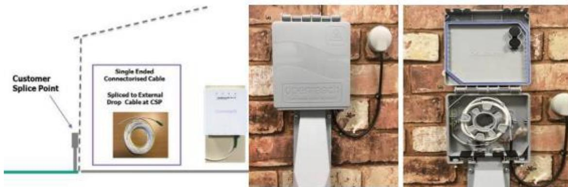
The external CSP is suitable for 80% of premises across the UK but cannot be used outside beyond safe working height or for certain types of building facia so Openreach have designed an internal CSP to use in these scenarios. It is very small and discreet by design and would be for use up to 2 metres from entry inside the premises
